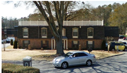
Versailles Apartments Demolished: 2013
